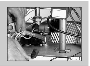
Removing the D.H.W. temperature sensor (N.T.C.)
